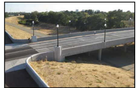
The new floodwalls will allow the bridge to remain open during a 200-year flood. Ornamental bridge lighting and vintage concrete barrier rails help improve bridge aesthetics.
