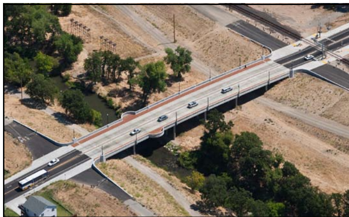
Completed project with architectural features and colors that match the environment and improve the overall aesthetics in the community.
