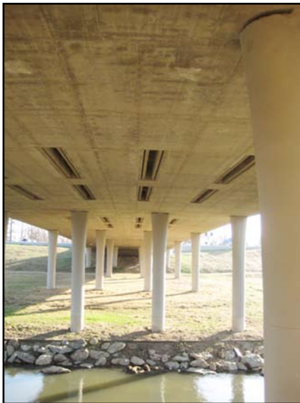
Permanent roosting habitat for bats was incorporated in the design of the underside of the bridge deck, providing distinctively upscale residences for 10,000 bats.
