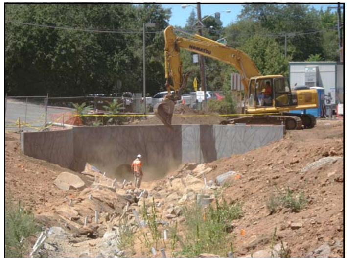
Retaining wall covered by black liner in first photo above, now visible, shows its architectural surfacing.
