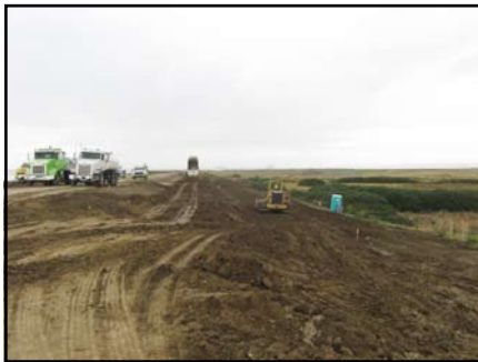
Construction of the landside setback levee.
