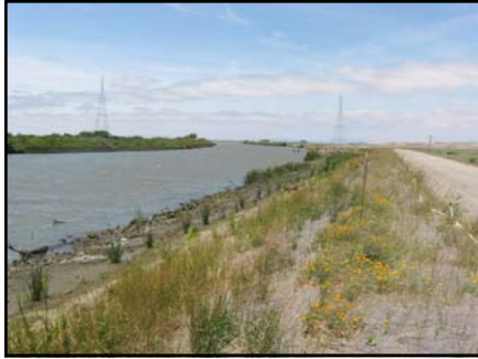
Setback levee habitat bench approximately 6 months after installation.
