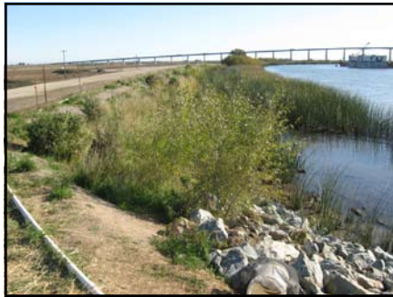
Setback levee habitat bench approximately one year after construction, showing lush vegetative growth on the intertidal bench and waterside levee slopes.
