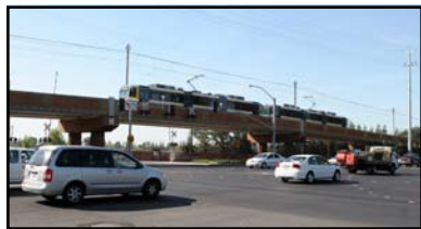
The Watt Ave./Folsom Blvd. Intersection after project completion.
