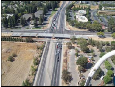
Aerial photo of structure during construction, just after erection.
