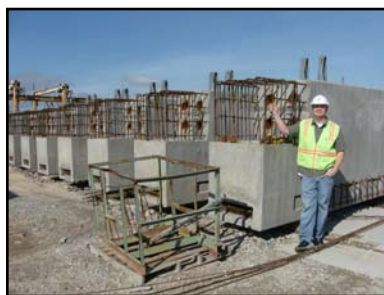
The precast concrete girders in the manufacturer's yard prior to site delivery and erection.
